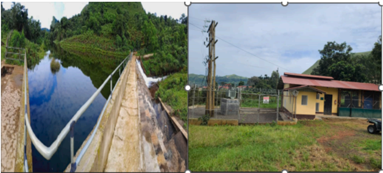
Fig. 2. Hydroelectric power dam and power station.
